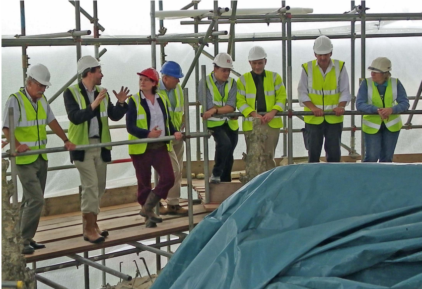
Stephen Oliver (2 nd left), church architect for the restoration project, with a group of visiting architects in the scaffolding tower above the roof of the apse
